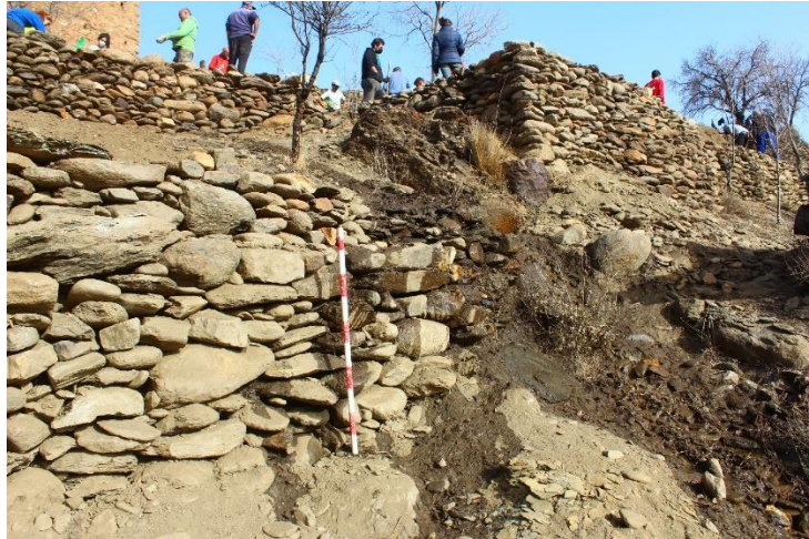
Figure 7. High dry stone terrace wall ( portillo or parata ) with a setback after reconstruction (source: MEMOLab)
