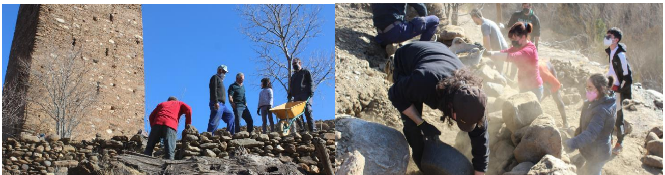
Figure 6a. Dry stone terrace wall ( portillo or parata ) reconstruction work (source: MEMOLab)
