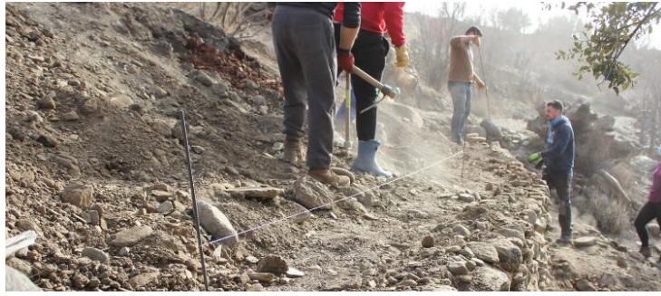
Figure 6b. Dry stone terrace wall ( portillo or parata ) reconstruction work (source: MEMOLab)
